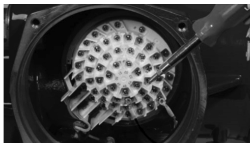
Figure 3.8 - Connecting network cable to terminal block
